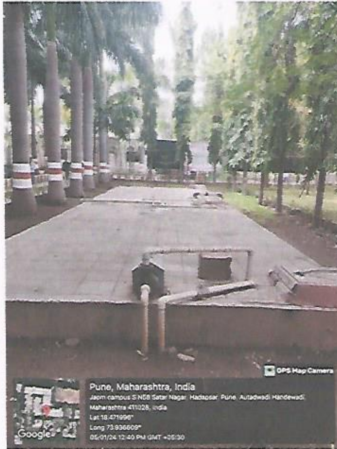
Construction of tanks and bunds
